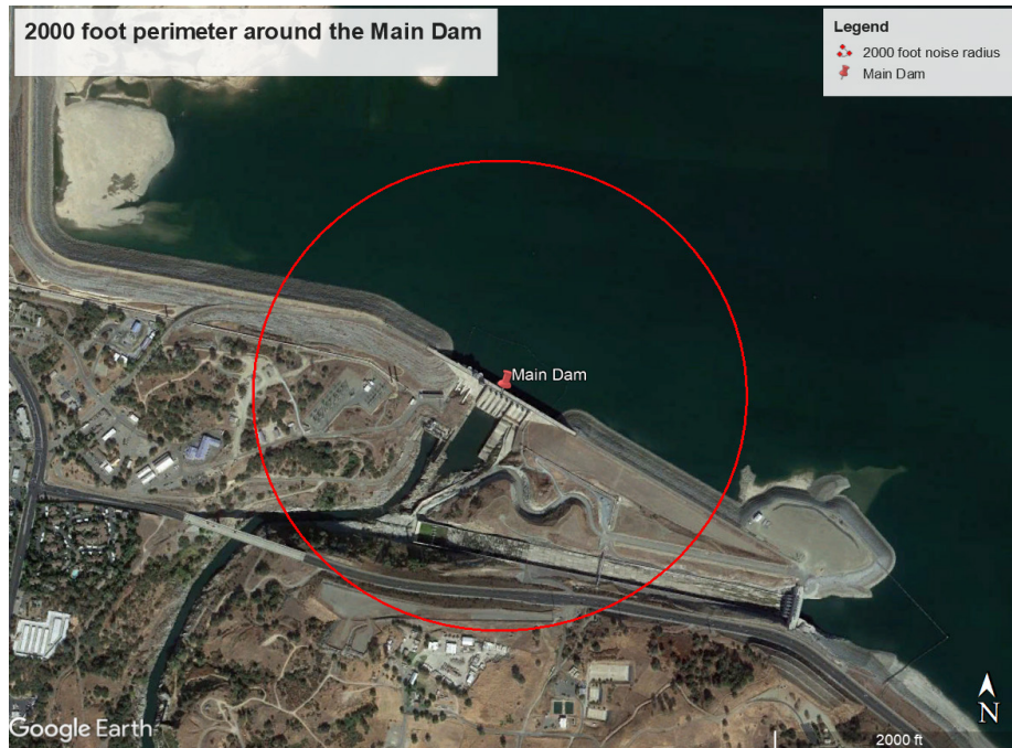
Figure 3-12. 2,000 foot noise buffer around the Folsom Main Dam.
